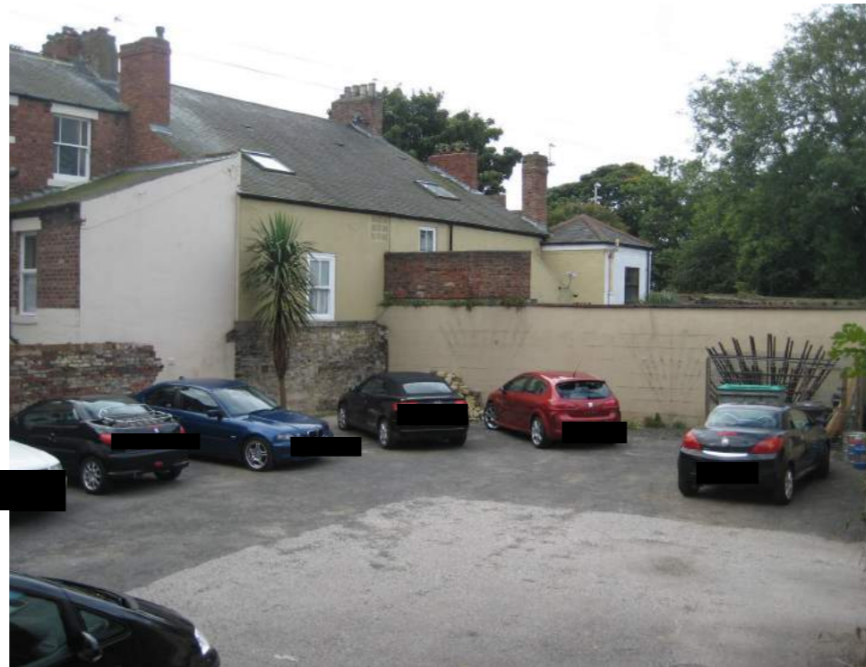
VIEW OF THE COURTYARD LOOKING WEST TOWARDS THE BOUNDARY WITH 2 AND 3 WESTOE VILLAGE
