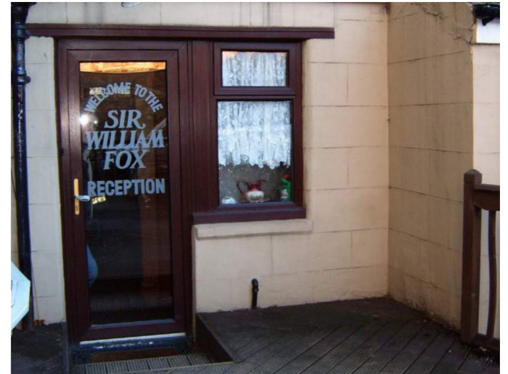
VIEW OF THE CURRENT ENTRANCE
