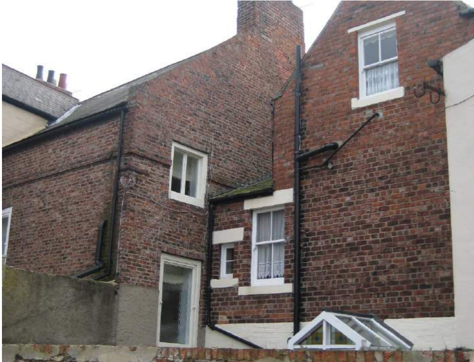
VIEW OF THE REAR AND SOUTH WEST SIDE ELEVATION OF THE MAIN GEORGIAN TOWNHOUSE AND ITS ABUTMENT WITH RED HOUSE
