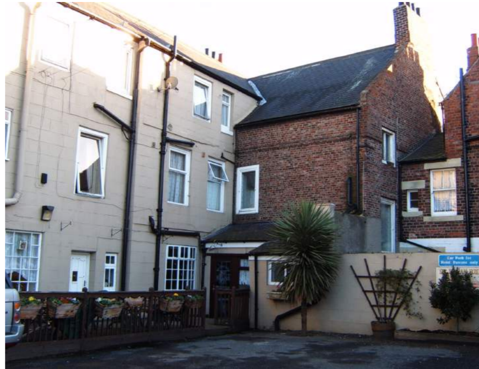
JUNCTION BETWEEN EARLY AND LATE GEORGIAN BUILDINGS
